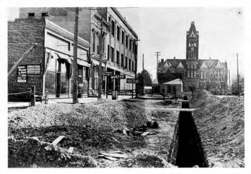
Photo from Geneva State Bank Laying steam pipes to heat courthouse and business houses (about 1910).
