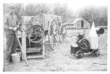
Cider press, powered by a portable 4-HP gasoline engine (about 1915).
